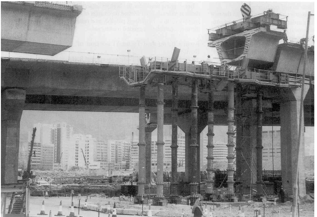
PHOTO 5.8 West Kowloon Expressway Viaduct, Hong Kong, during construction, comprising 4.2 km dual three-lane causeway connecting Western Harbor Crossing to new airport (courtesy Institution of Civil Engineers, London, and [5]).
