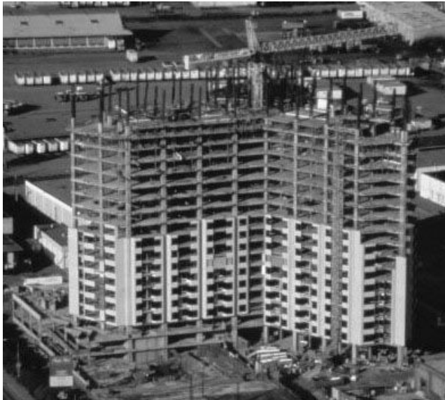
PHOTO 4.1 A 30-story reinforced concrete building under construction. The Pacific Park Plaza is one of the largest reinforced concrete structures in the San Francisco Bay area. It survived the October 17, 1989, Loma Prieta earthquake without damage. Instrumentation in the building recorded peak horizontal accelerations of 0.22g at the base and 0.39g at the top of the building (courtesy of Mr. James Tai, T.Y. International, San Francisco).
